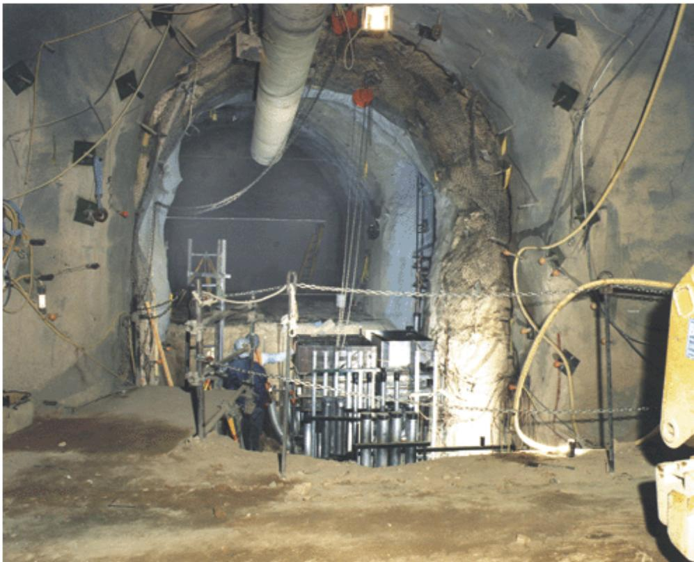
One of two experimental alcoves in the 102 minicomplex during construction. Workers are installing the utilities required to stage and diagnose subcritical tests.
